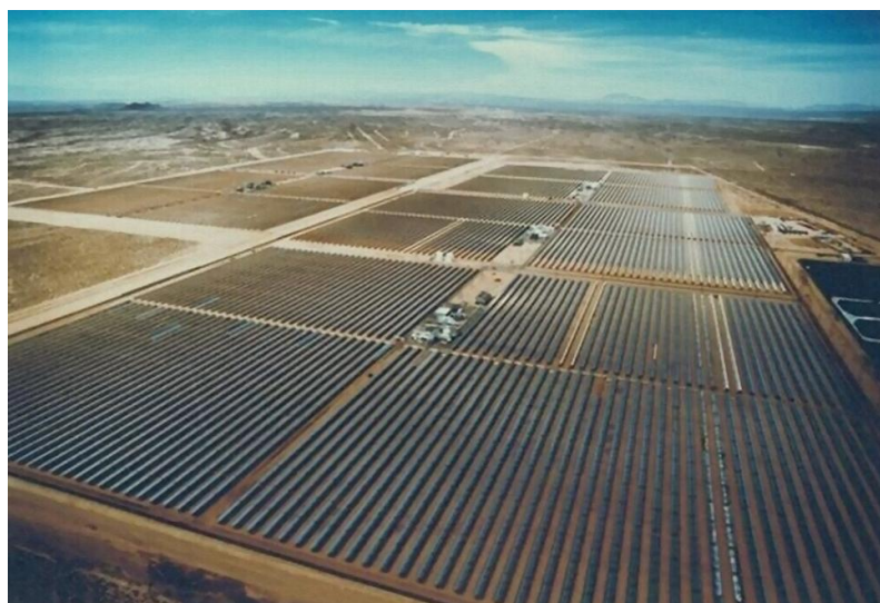
Figura 2.11: Centrales SEGS III a VII, Kramer Junction, California.
