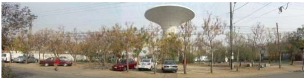
Vista norte_ Calle Petrohue
