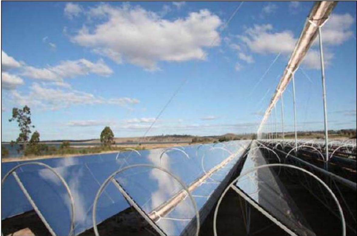
**Figura 19: “Planta Colectores Lineales Fresnel” [16]**
