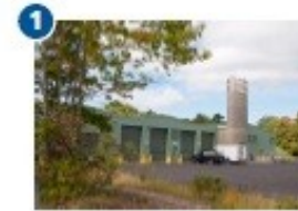
The woodchips are delivered by trucks, each carrying 30 tons of the biofuel, and stored in a 17,500-cubic-foot bunker that can hold a week's worth of fuel. One ton of woodchips is the equivalent of 61 gallons of heating oil.
