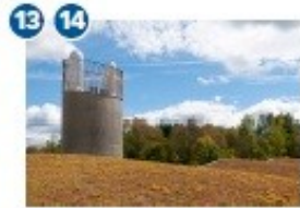
The 48-foot chimneys disperse emissions into the prevailing winds, reducing ground-level impacts to nearly zero.
