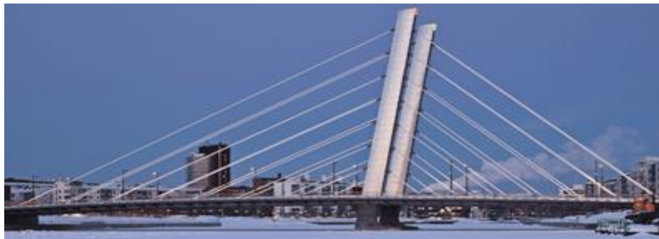
Figura 2.12: Crusell Bridge (WSP, 2010)
