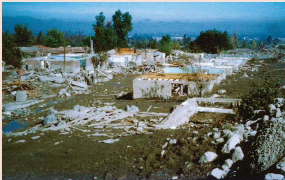
FIGURE 4 Devastation resulting from the flash flood of 3 May 1993 in Macul watershed. (Photo by Francisco Ferrando)
