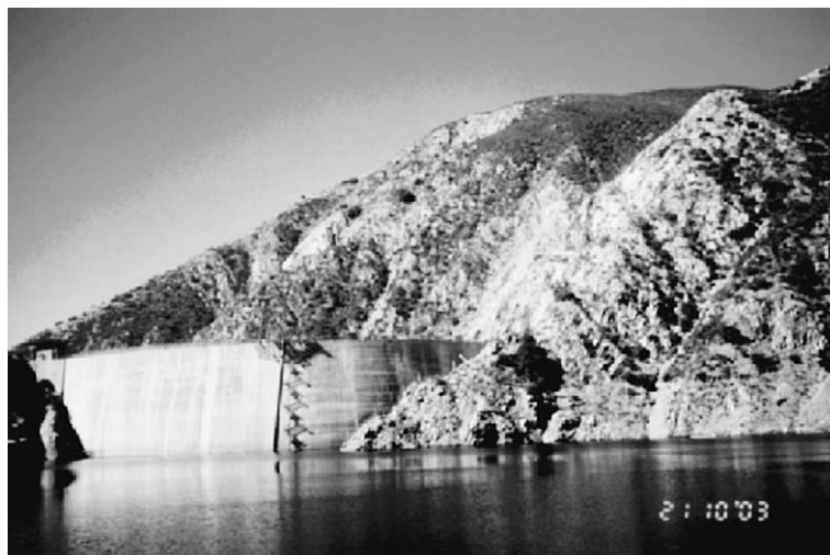
Fig. 2. Pacoima dam and reservoir, and rock mass of the right dam abutment.
