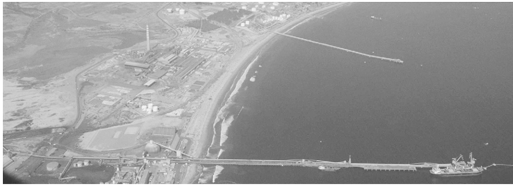
(a) Aerial view looking south.
