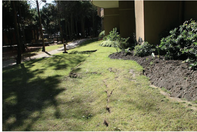
Figure 5. Soil depression along ocean-facing side.
