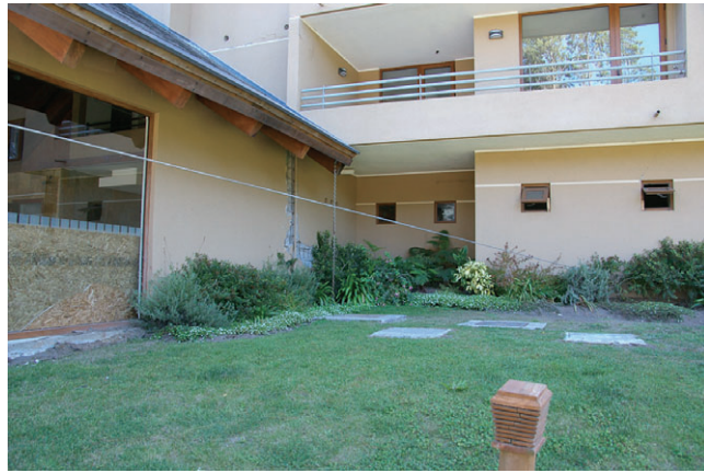
Figure 13. First floor wall along gridline 22.
