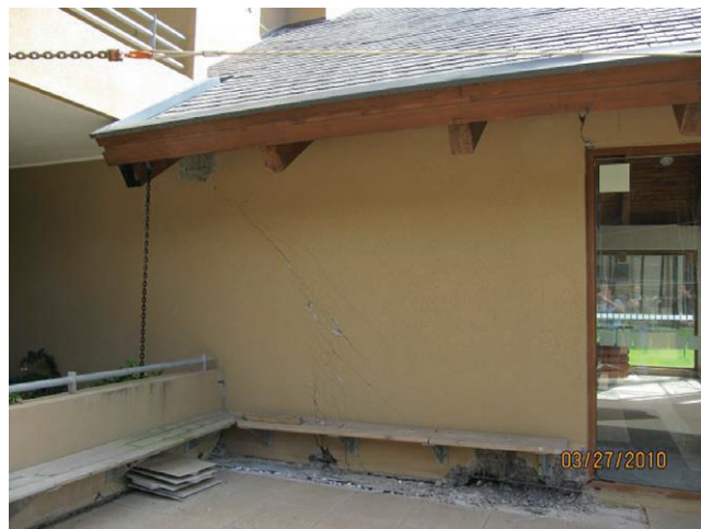
Figure 12. First floor wall along gridline 15.
