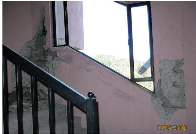
Figure 22. Interior view from stairwell.
