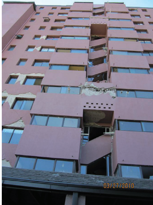
Figure 20. Diagonal stairwell elements along height.
