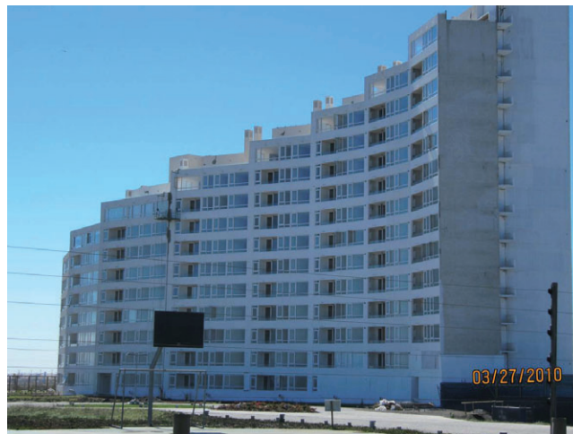
Figure 25. Olas building in San Pedro de la Paz.
