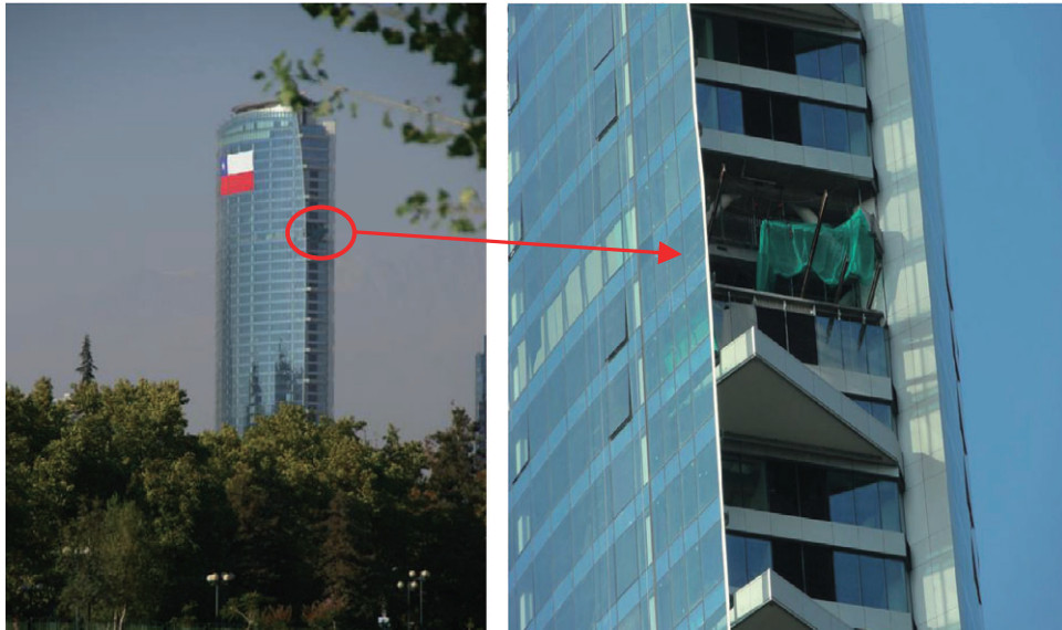
Figure 8. The Titanium Tower, local cladding damage.
