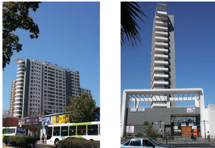
Figure 19. Views of the Emerald Building.
