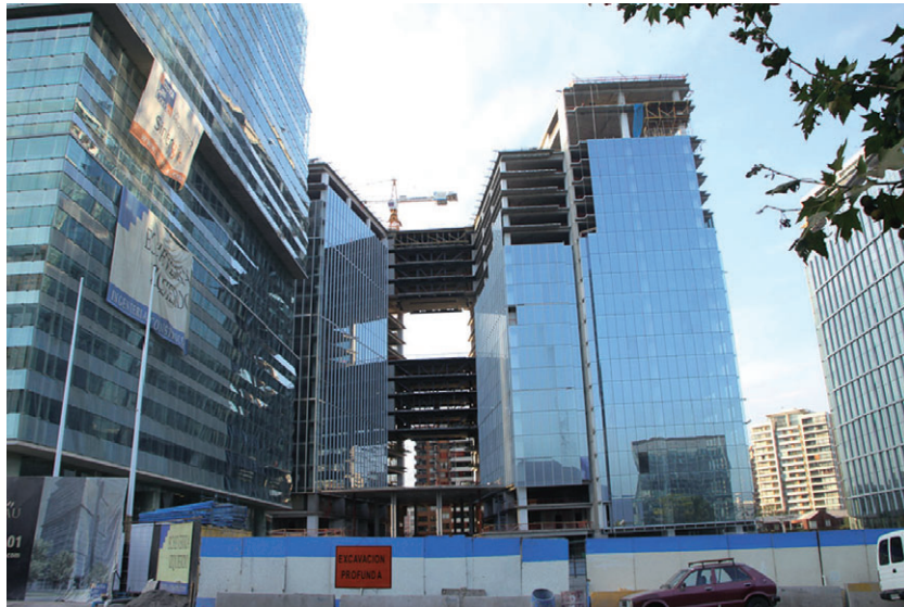
Figure 13. The Echeverria Izquierdo Building.
