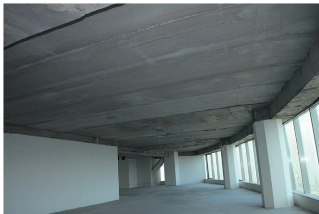
Figure 9. The precast columns and floor system implemented at the Titanium Tower. (a) Connection of damping brace to the floor above. (b) Damping system at the middle of braces. (c) Passing of the damping brace through intermediate floor.
