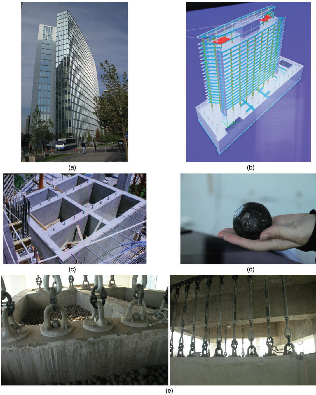
Figure 12. The Parque Araucano building and its TMD systems. (a) Post-earthquake view from outside. (b) Computer model with TMDs shown in red. (c) TMD box during construction. (d) Size of metal balls filling the TMD cavities. (e) Completed and filled TMD hanging from the roof above.
