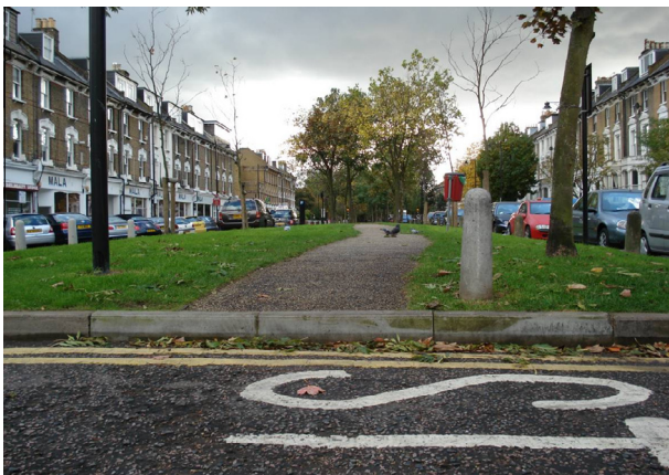
Fig. 1.3. Example of discontinuity of access in pedestrian pavement.
