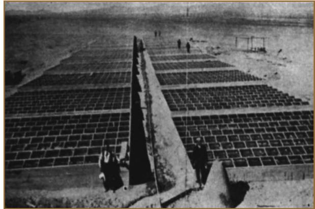
**figure 2.** The first solar energy desalination system in Chile, 1872 (source: J. Hirschmann).
