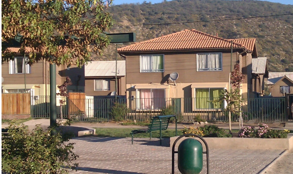
Figure 1: Houses in Casas Viejas are relatively homogenous in their appearance, however ceramic tiles are used for the affordable house and corrugated metal for social housing.
