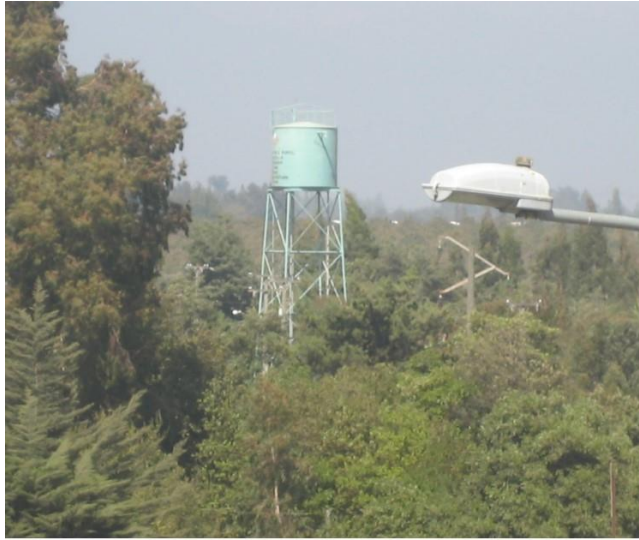
Figura 16: Agua Potable Rural
