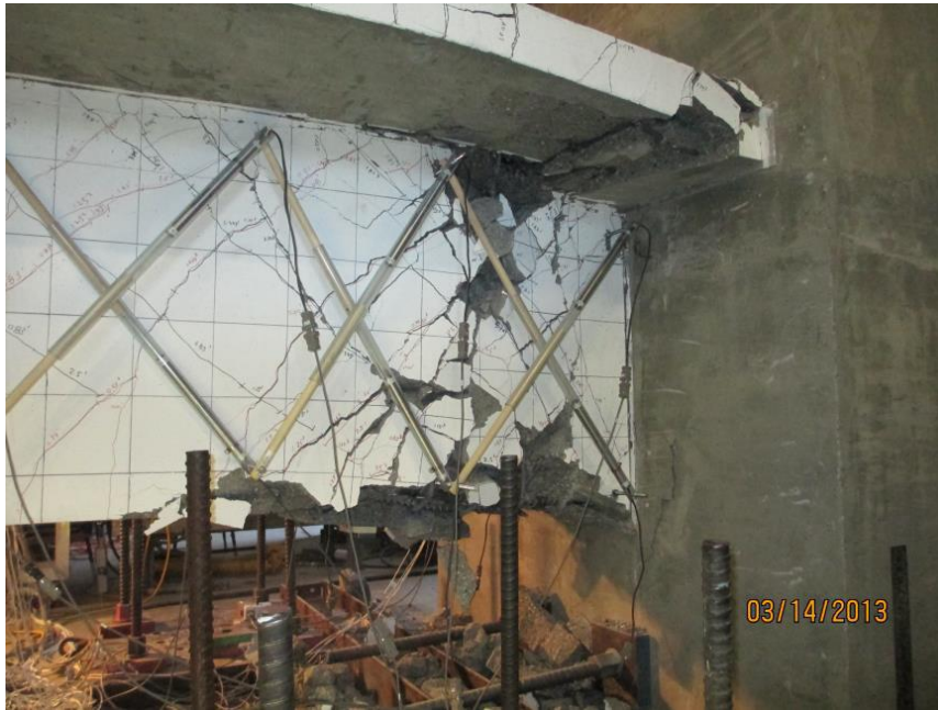
Figure 3.20: Early plastic hinge with separation of the top slab (Specimen 7), (Lemnitzer et al., 2013).
