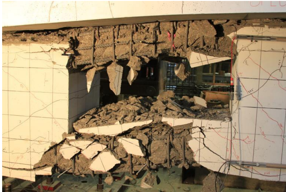
Figure 3.15: Opening section at test termination (Specimen 1), (Lemnitzer et al., 2013).
