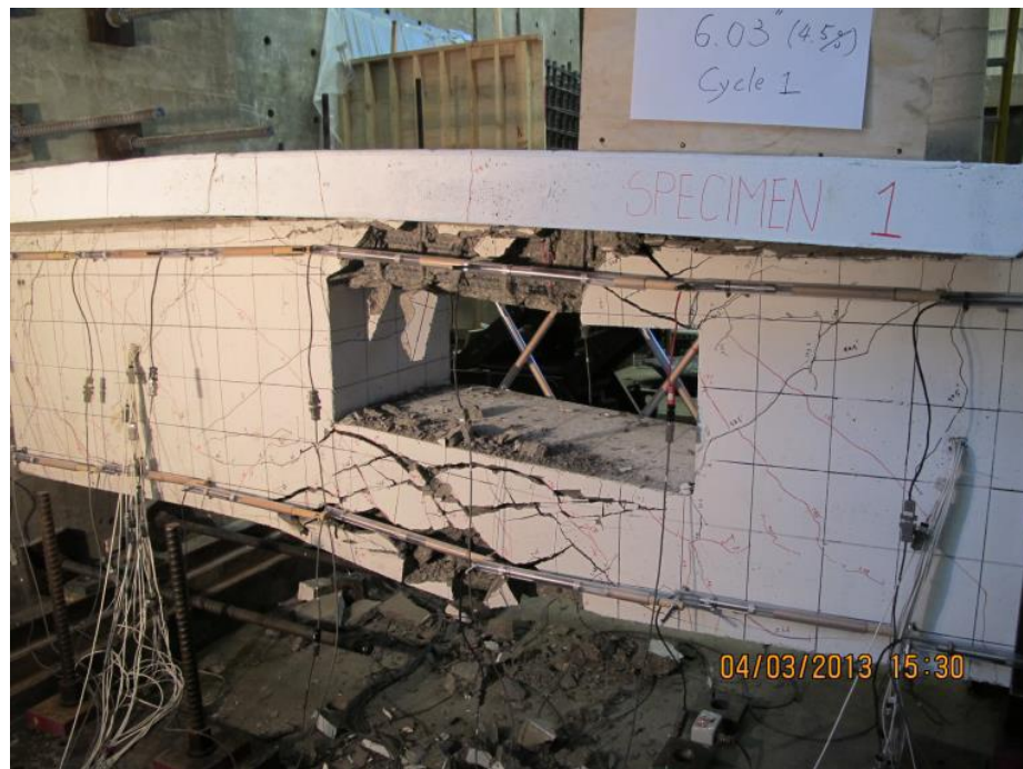
Figure 3.14: Plastic hinge at 4.5% drift level (Specimen 1), (Lemnitzer et al., 2013).
