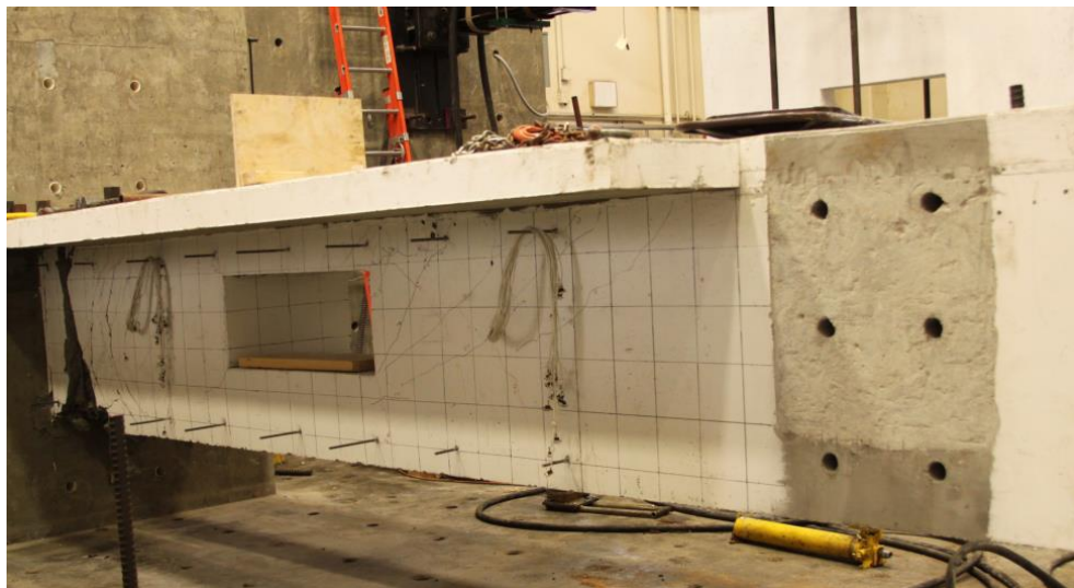
Figure 3.19: Undamaged opening at Specimen 6 after test completion and plastic hinge at the far left of the picture, (Lemnitzer et al., 2013).
