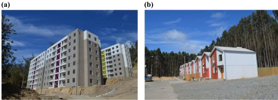
Notes: (a) Quinta Gaete, constructed on a steep slope; (b) Villa Verde, surrounded by forestland
