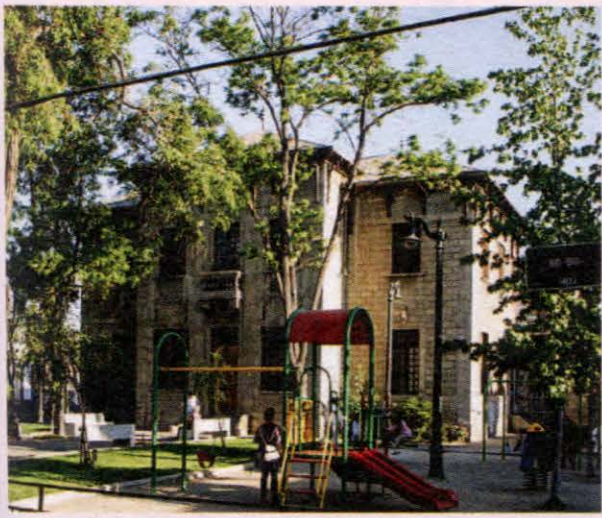
The square and building of the Workers' Building Societies promote a barrio identity: Huemul housing development, Santiago. Larraín Bravo (1911).
