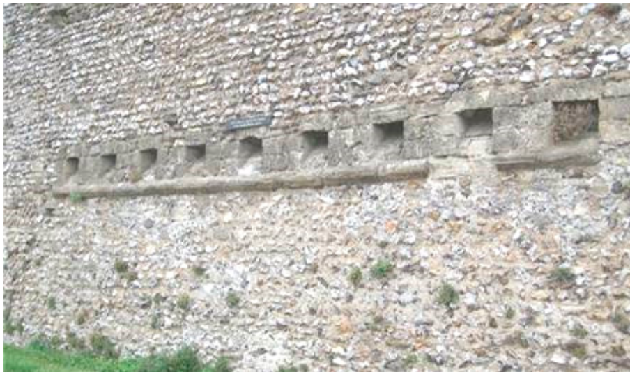
Figure 37. The latrine chutes on the enclosure walls at the Portchester Castle–Benedictine Priory ca. 11th c. [79–83]. The resemblance to the lavatory at the tower of Sinai monastery dated in the 6th c. (Figure 27b) is obvious.
