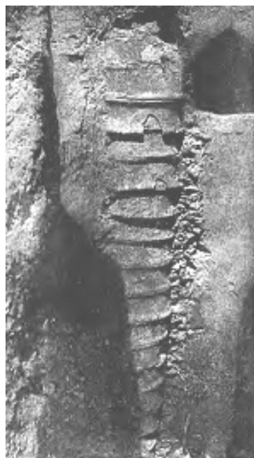
Figure 4. Clay baked pipes of a vertical pit at the city of Adab (second half of third millennium BC) (adapted from [20], p. 346).
