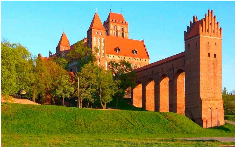
Figure 39. Kwidzyn Castle Poland. On the right the high detached lavatory tower. On the left, behind the trees, the short detached lavatory tower (Panoramio, Knapczyk, 2015) [79–83].
