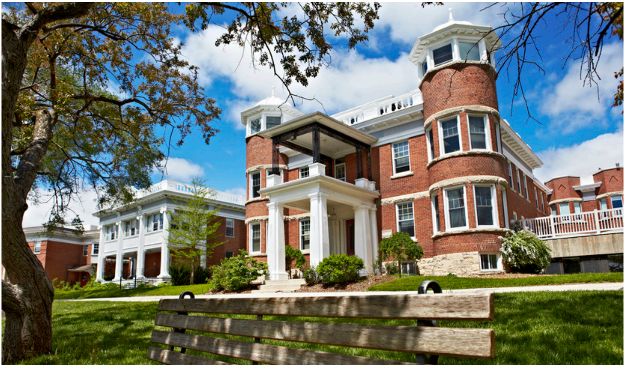
Figura 118: Fachada principal del Homewood Health Centre. Fuente: http://www.homewoodhealth.com
