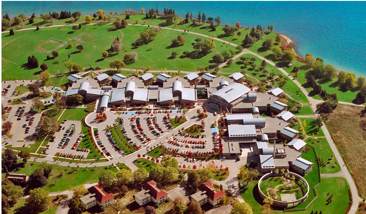
Figura 109: Vista aérea Whitby Mental Health Centre, 2005. Fuente: http://www.flickr.com , de Ontario Shores Centre for Mental Health Sciences
