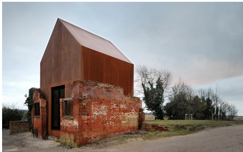
Dovecote Studio, Haworth Tompkins Architects, Suffolk, (Fuente: http://www.haworthtompkins.com/ )
