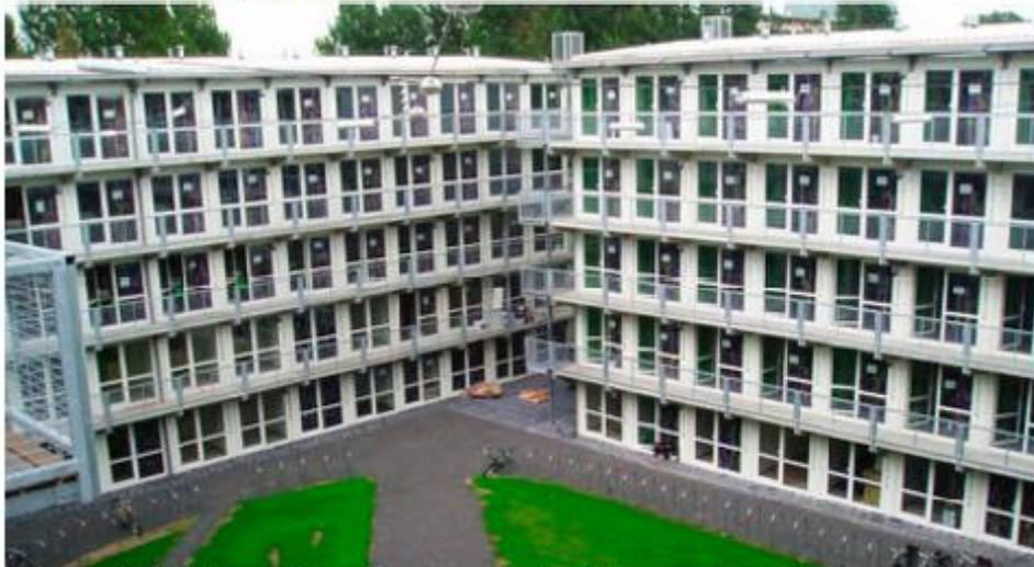
Creating affordable housing for students is a particular challenge within the Dutch system because its complex point-based system of rent control does not allow raising rents to levels needed to support development costs. De Gooijer thought used containers could be converted to student housing at a low enough cost to be supported by controlled rents.
