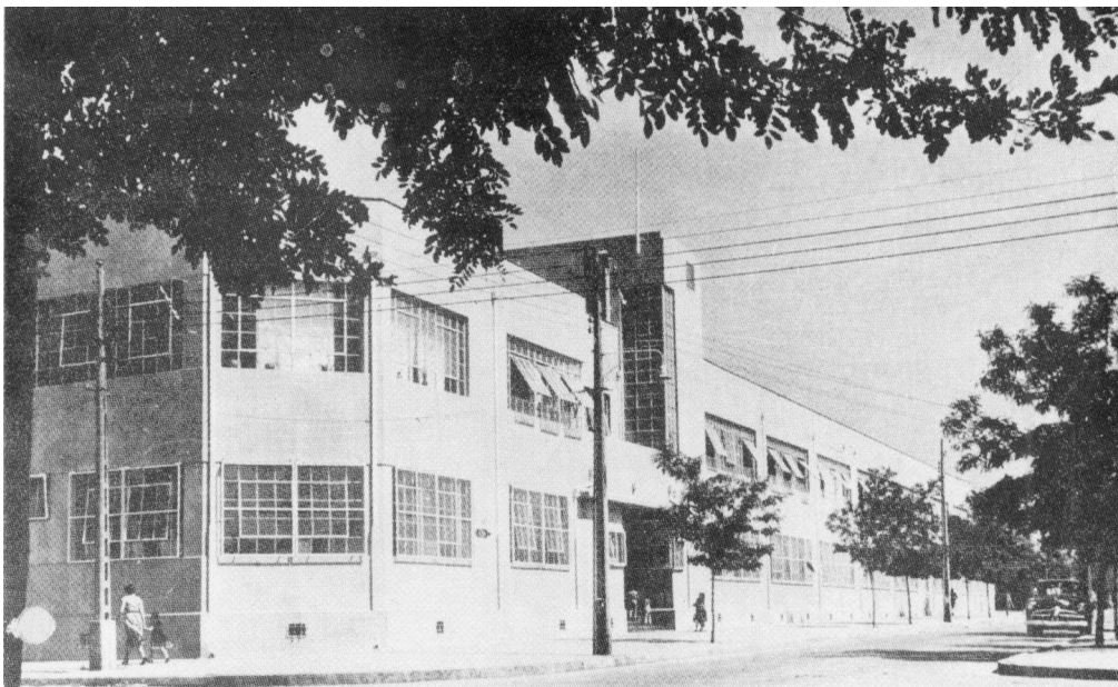
Figure 7. Girls school in Santiago, School D-24, 1938; the first school built by the SCEE (source: Sociedad Constructora de Establecimientos Educativos, 50 Años de Labor , 1987).
