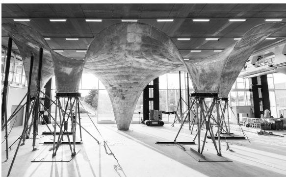
39. NEST HiLo shell roof, cascara en hormigón, Block Research Group, 2017 39. NEST HiLo shell roof, guscio in calcestruzzo, Block Research Group, 2017
