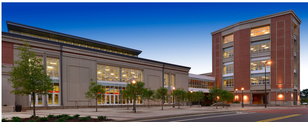
Figura 4.9 Exterior Rec & Wellness Center, Auburn University. Fuente : www.hok.com
