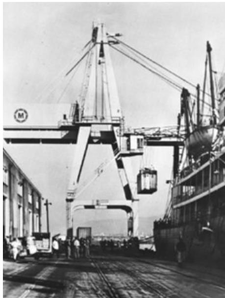
*Figura 2.8: Primera grúa de STS desarrollada. (Fuente: Development of design of ship to shore container cranes)*
