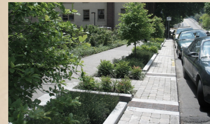
Southwest Montgomery Green Street Portland, EEUU.
