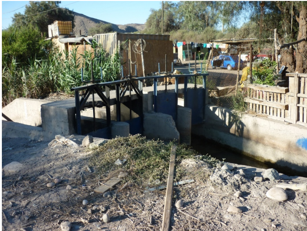
Figura 3.8: Obra terminal – Km 10+788
