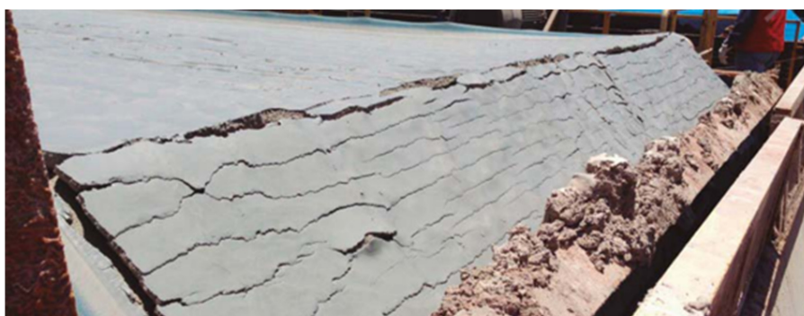
Figure 9. Filtered Tailings Technology—Tailings Filters at Mantos Blancos Mine Chile [11].
