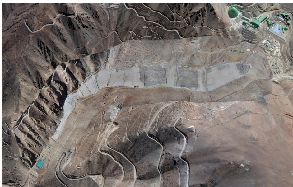
Figure 10. Sand Stack TSF (Cycloned Sand Tailings) SSSTT—Caserones Mine, Chile [18].
