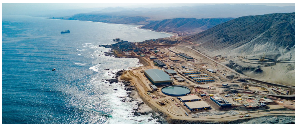
Figure 15. Escondida Mine Sea Water Desalination Plant, Chile [44].
