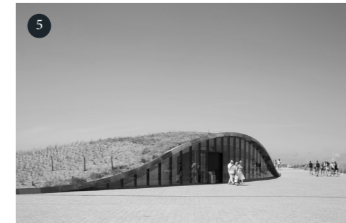
Parque Subteraneo Katwijk Royal Haskoning DHV Architects
