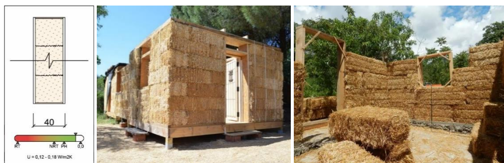
Figura 8-9 Sistema Nebraska (Taller Karuna ®, 2015) (CONSTRUPAJAARGENTINA, 2015)
