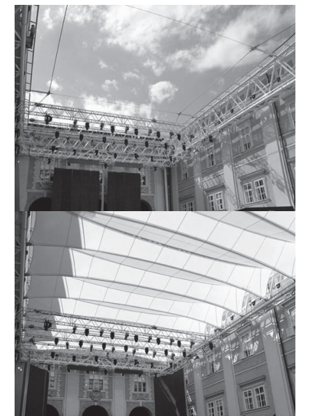
Método de Integración, Techo retráctil Residencia Salzburgo. Fuente: Kugel Architekten, Obtenido de https://www.kugel-architekten.com/content.php?n=1&d=24#:~:text=Assembly%20%5B12%5D-,Re-tractable%20roof%20for%20the%20Salzburg%20Festival%2C%20courtyard%20of%20the%20Salzburg,(U-NESCO%20World%20Heritage%20Site).
