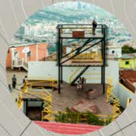
Mirador 70 maan architecture
