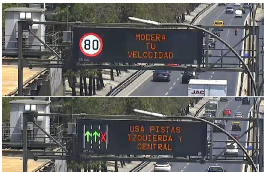
Figure 2. Variable messaging panels “Moderate your Speed” and “Use left and center lanes” on the Autopista Central.
